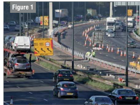
Figure 1 Steel barrier replacement works – lane closures and traffic management
