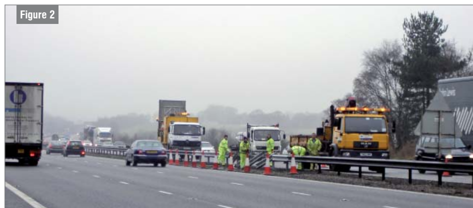
Figure 2 Repairs to steel barrier following minor impact
