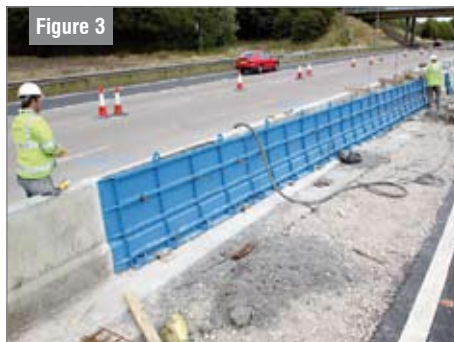
Figure 3 In-situ casting at bifurcation
