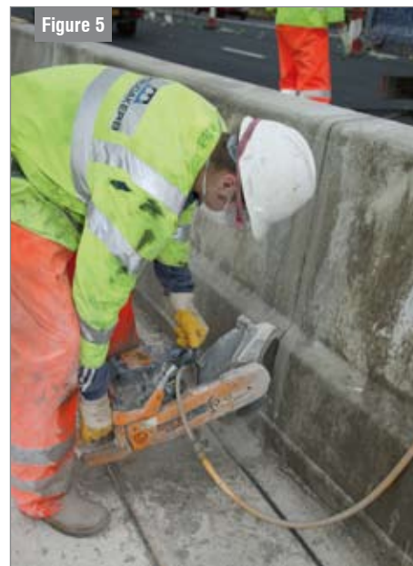
Figure 5 Saw-cutting CSB
