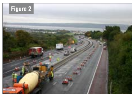
Figure 2 Barrier construction
