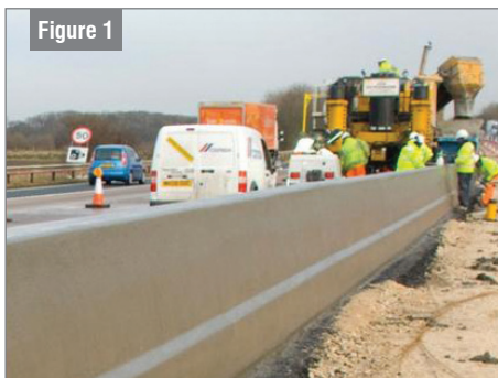
Figure 1 Traffic management during construction
