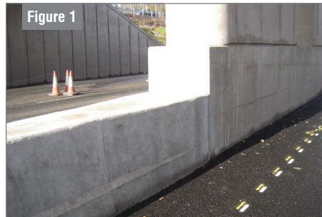
CSB transition to bridge pier
