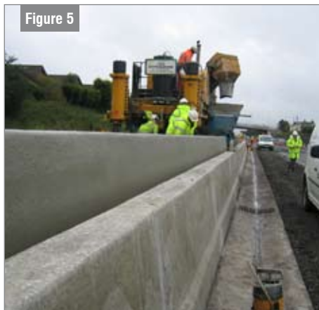
Weep holes to drain area in between barriers
