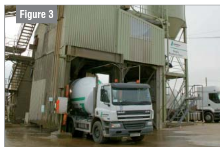
Dedicated concrete plant
